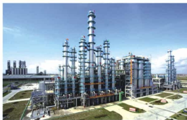
Industrial control system
