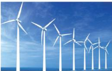
Wind energy system
