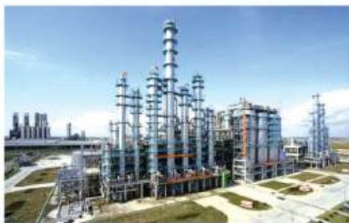
Industrial control system
