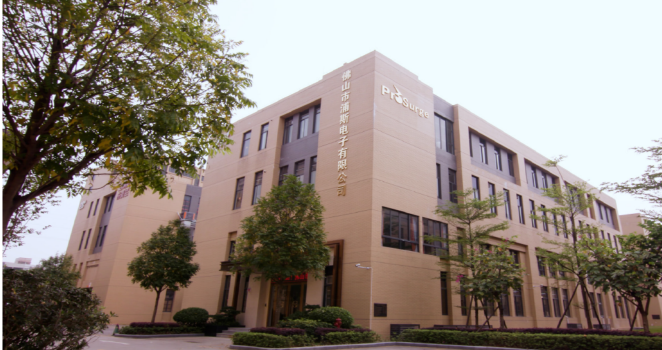
Prosurge Electronics Co., Ltd - Foshan, China
